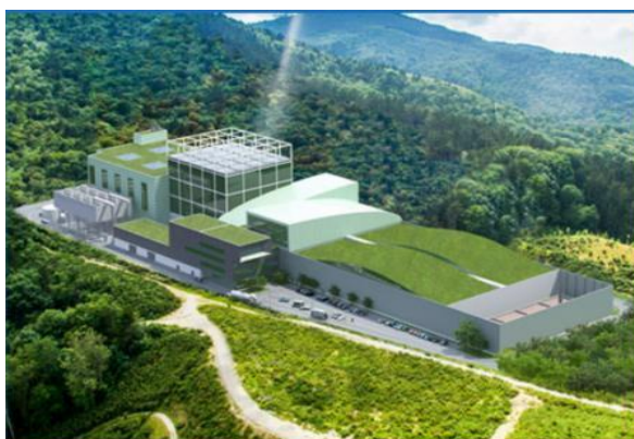
Incineration ,for Steelmuller in Zubieta ( Spain ), 2017 ONGOING
