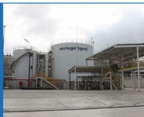
Marpol Treatment plant , SERTEGO ( TANGER), 2016
