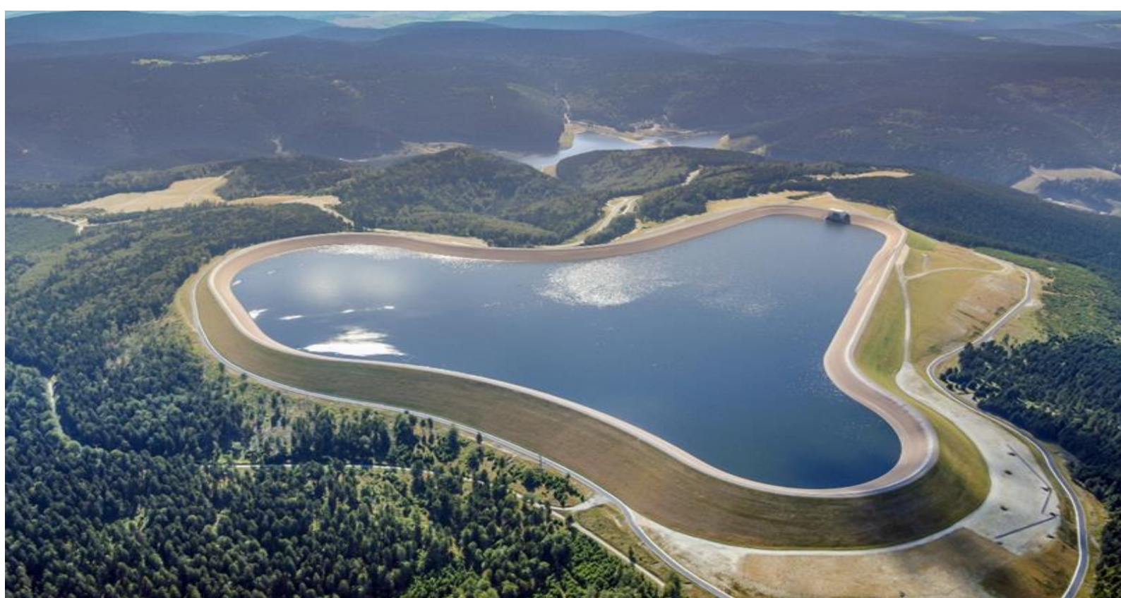
Fig. 1 An aerial view of the Goldisthal Pumped Storage Station, the largest hydroelectric power plant in Germany and one of the largest in Europe
