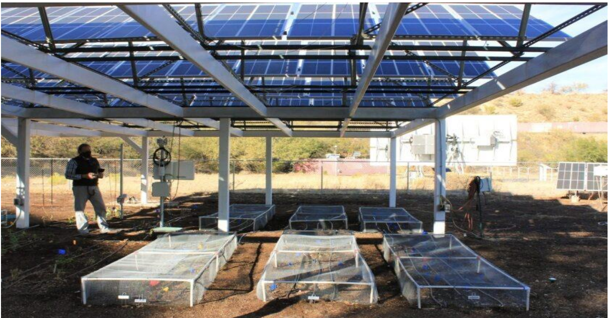
Solar Farms can be built eight feet off the ground to enable food production underneath also saving 40% on water usage and upto three times crop growth.
