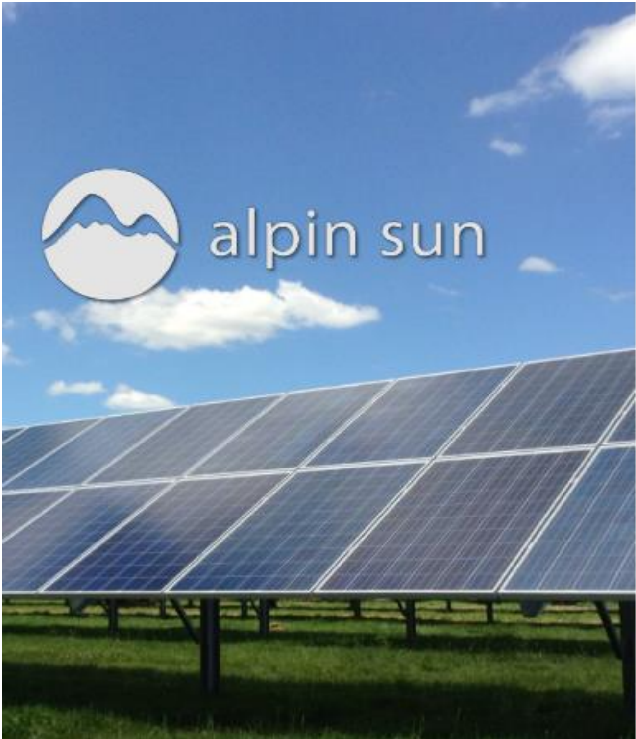
25MW Solar Farm site at Nakuru
