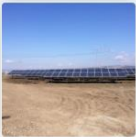
Reci, Covasna, RO 2,133 MW
