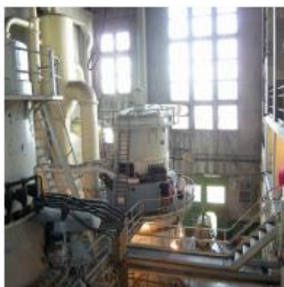
E86152 Innovest IBAE, Kuala Lumpur, Malaysia Fuel: Heavy oil (3-6% S) oil fired IBAE boiler
