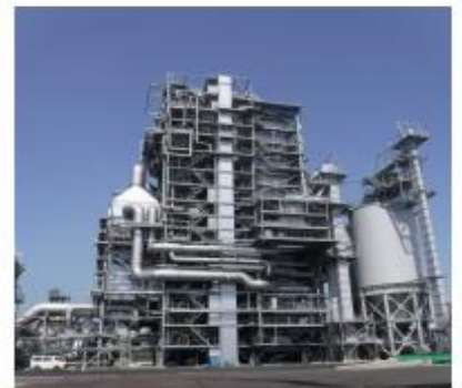
E84104, Eastern Illinois University, Charleston, IL Fuel: Coal fired chain grate boiler
