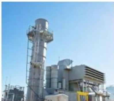
Installation of Westinghouse 501-F Gas Turbine
