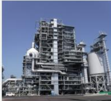
Gemma Power Systems, Monroe, GA Installation of Westinghouse, 50-F Gas Turbine
