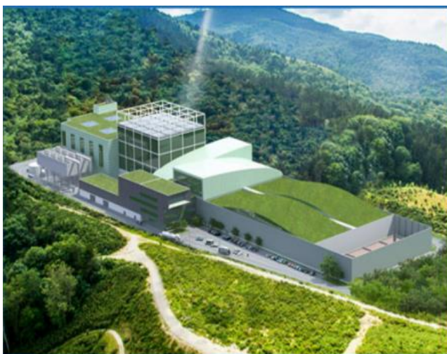
Incineration ,for Steelmuller in Zubieta ( Spain ), 2017 ONGOING
