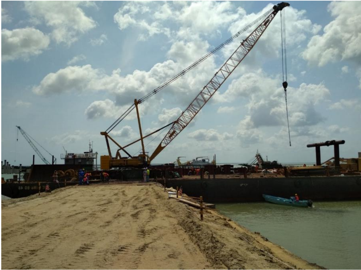
Photo 2: Port construction works
