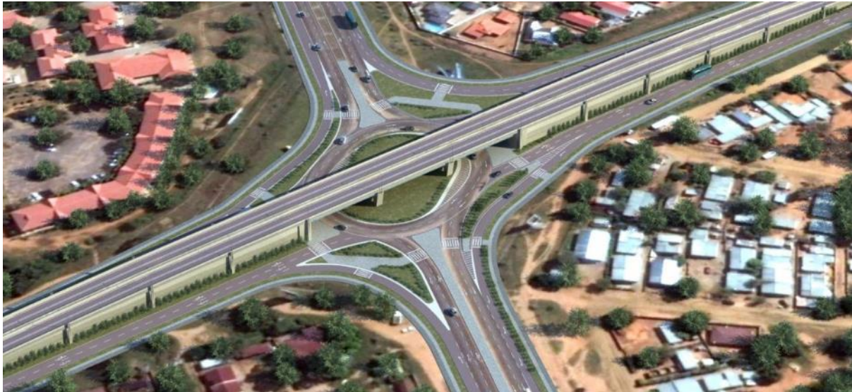
Figure 18: Visual image of diamond type interchange with roundabout at the ground level and provision for NMT facilities
