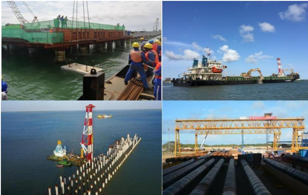
Photo 21: Port construction works in progress
