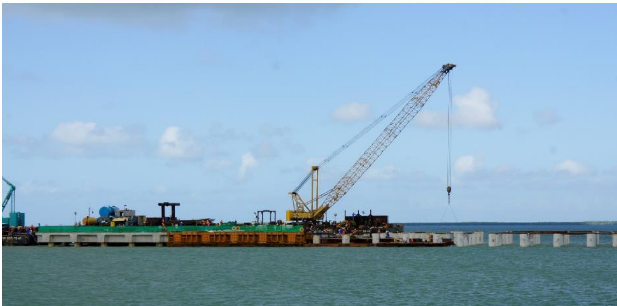
Photo 9: On-going construction works for the first berth
