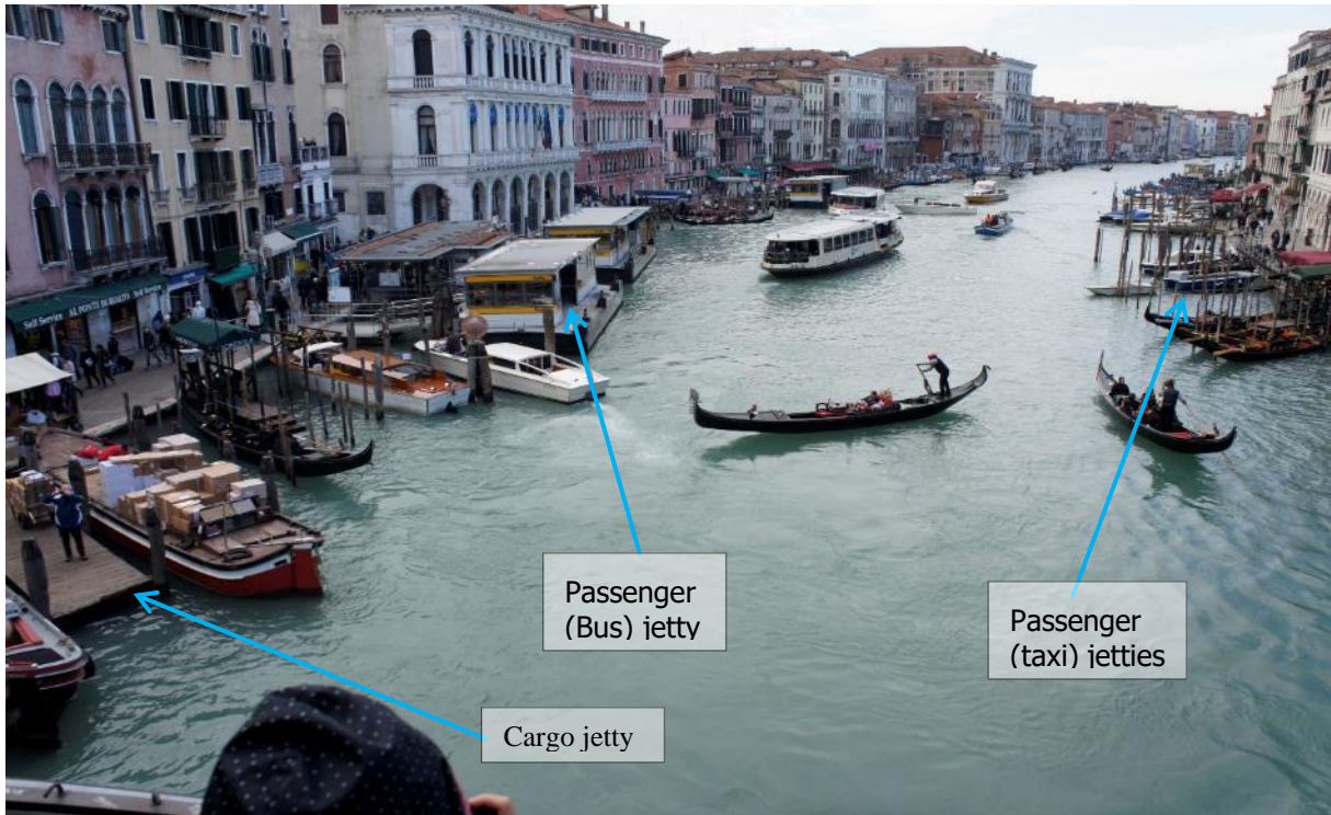
Photo 30: Example of multiple different type jetties
