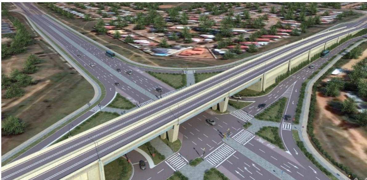
Figure 17: Visual image of a diamond type interchange with provision for NMT facilities on ground level
