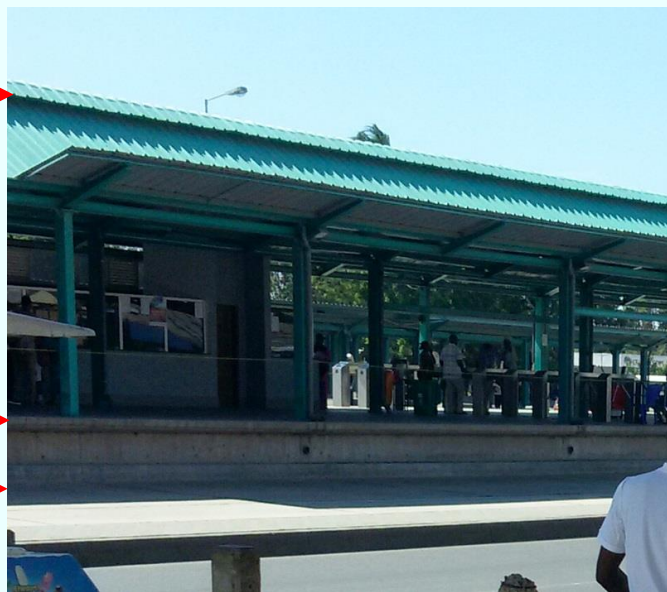
Photo 34: Example of BRT Platform with raised floor for exclusive use of BRT passengers (DAR)
