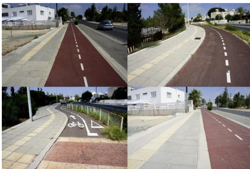
Photo 33: Combined Pedestrian-Cycling with differentiated materials and clear marking
