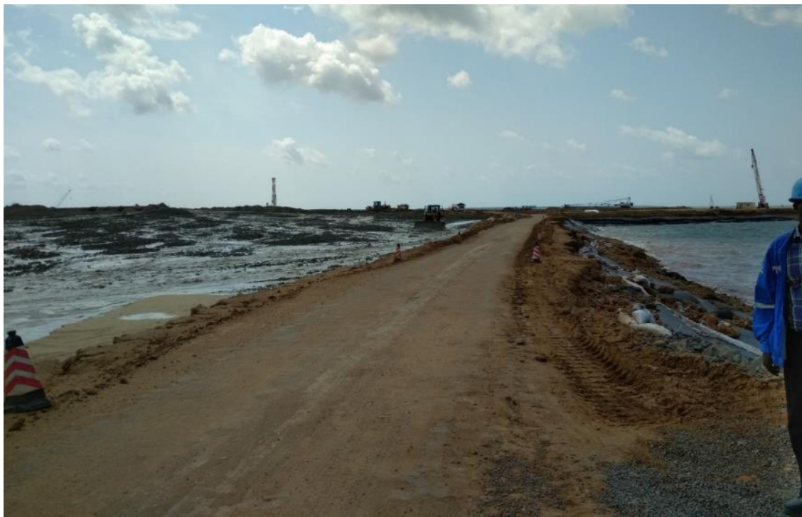
Photo 3: Causeway leading to port construction work site for initial 3 berths
