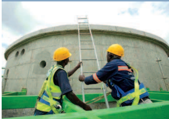
Photograph: Tropical Power
