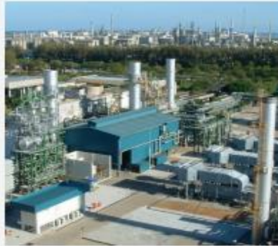
PG&E National Energy Group, Bowling Green, OH 50 MW Power Plant - Peaking Facility, 2 - GE Frame 5
