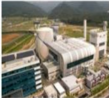
Combined heat and power plants
