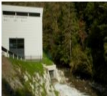
Small hydro power
