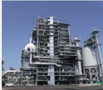
Gemma Power Systems, Monroe, GA Installation of Westinghouse, 50HF Gas Turbine
