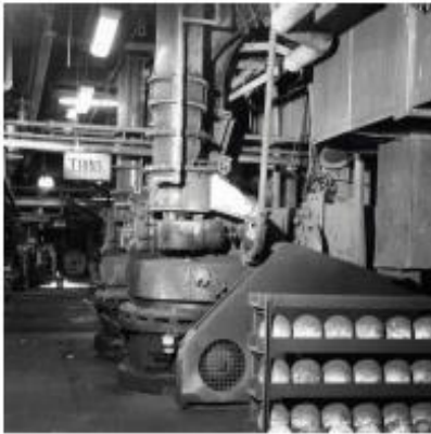
E87032 Montgomery County Incinerator Plant, Dayton, OH Fuel: Trash incinerator chain grate CE boiler
