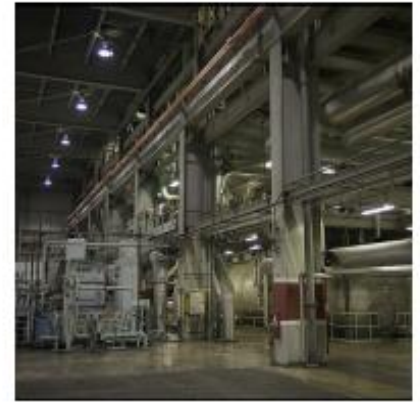
E86070 Union Carbide Corp., Charleston, WV Fuel: coal fired chain grate boiler #4
