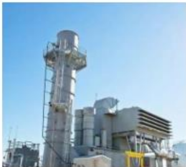
Installation of Westinghouse 501-F Gas Turbine
